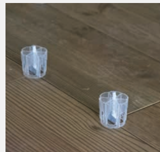
T-shaped leveler installation.
