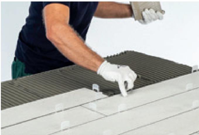
disposable clips installation
