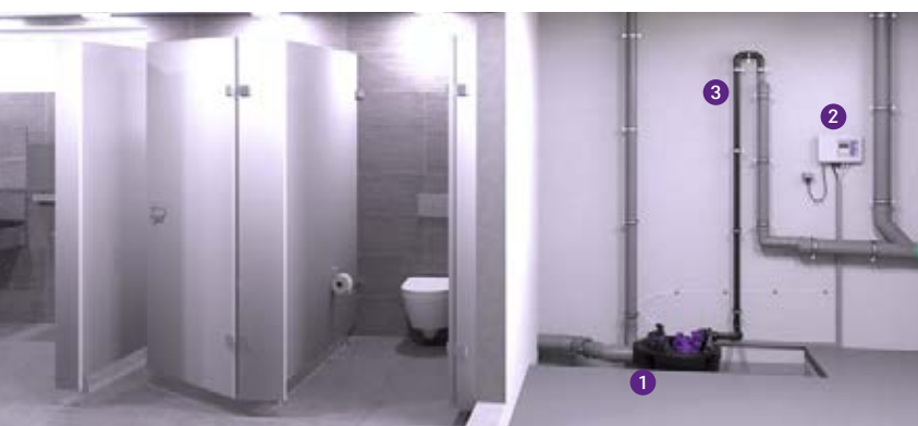
① Lifting station ② Control unit ③ Pressure pipe
