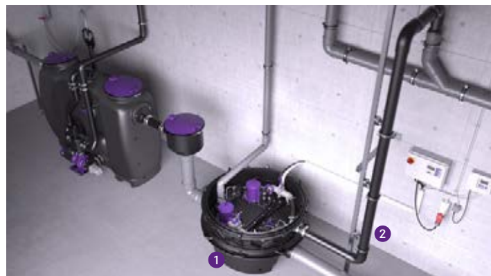
1 Hybrid lifting station 2 Pressure pipe
