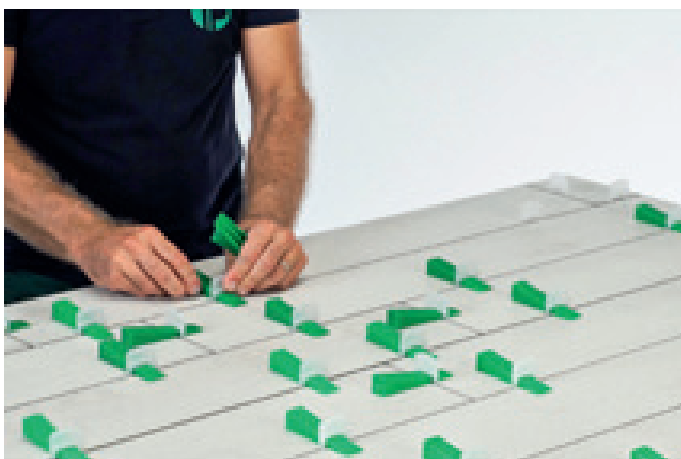
levelling wedges insertion
